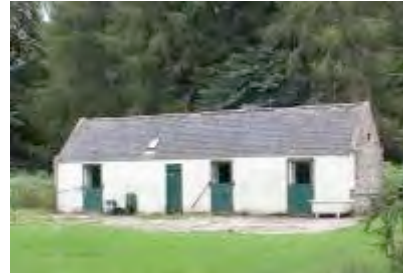
Fig.3 – former stable block
